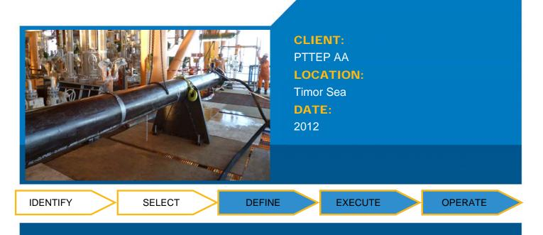
Following the Montara well blowout, concerns were raised about the potential for accelerated internal corrosion of the carbon steel risers. As part of the Montara WHD Platform Riser Inspection Campaign, Linch-pin was engaged by PTTEP AA to design pig and Ultrasonic Testing (UT) tool launchers and receivers to assist with the riser inspections.
