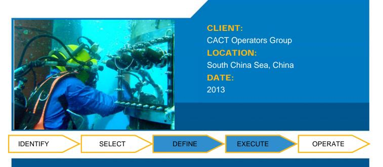
CACT was faced with the issue of subsea fatigue cracks in some Jacket joints on a platform in Bohai Bay, China. CACT wished to engage Neptune and their underwater weld repair technology but needed expert advice and management support while the technology was prequalified and the equipment mobilised to China.
